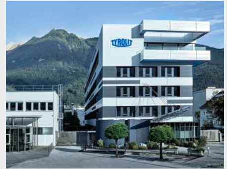
Tyrolit headquarters in Schwaz (Austria)
